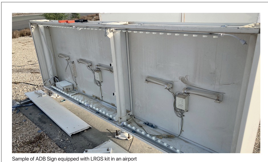
Sample of ADB Sign equipped with LRGS kit in an airport
